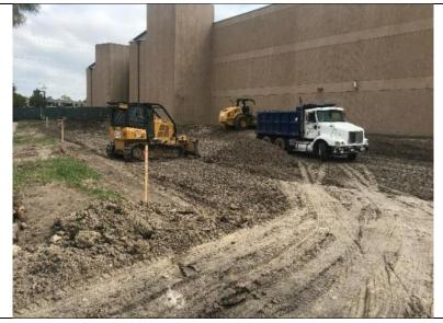
Select fill is being imported to the site and compacted in the existing detention pond basin.
