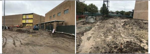
Concrete sidewalks and asphalt paving have been demolished. Underground storm sewer and manhole work is on-going
