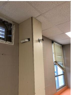
Old HVAC units have been removed, opening up the classrooms. Picture shows the patching of the wall and louver that remain to be worked on.
