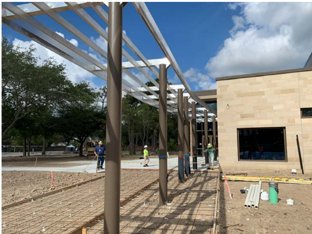
Forming Sidewalk and Bus Drop Off Canopy
