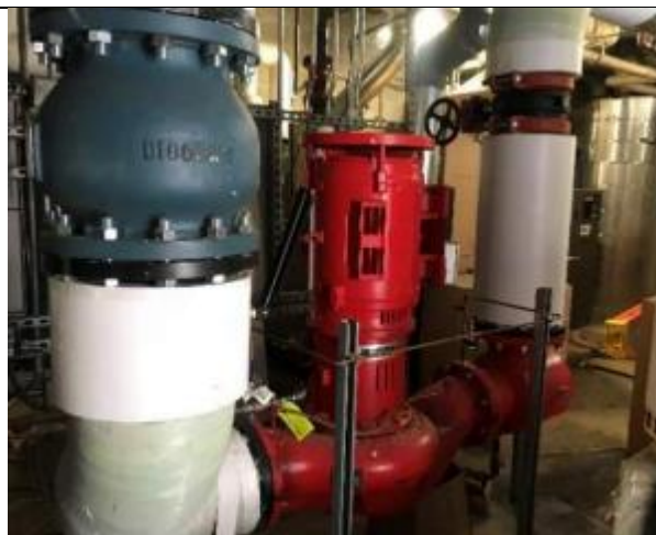
Hydronic pumps have been installed and connected to the piping runs.
