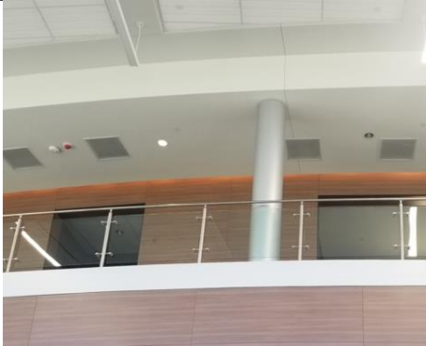
Column wraps have been installed at balcony.
