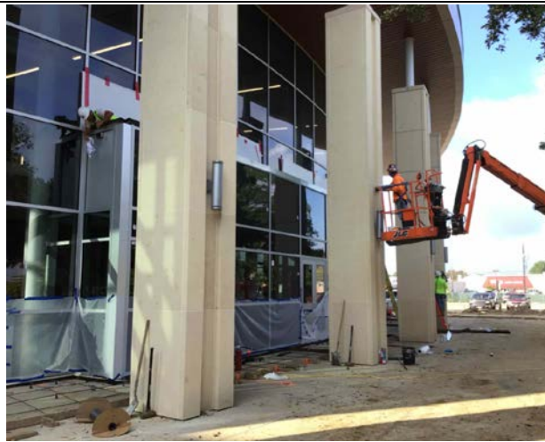
Exterior stone columns progressing with sealant.
