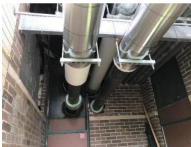
Main hydronic piping has been routed from chillers to the main mechanical room & insulated.
