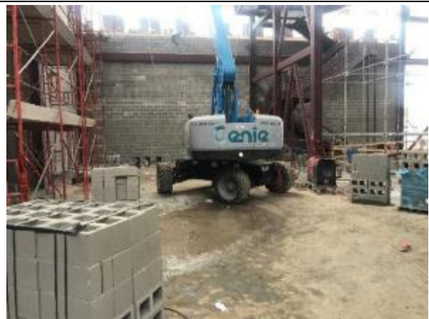
CMU is being placed along the Auditorium southwest wall area.
