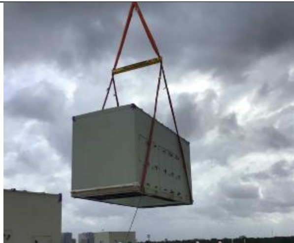
The new RTUs were craned lifted into place on the roof.
