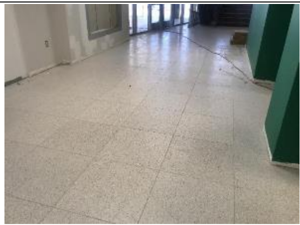
Terrazzo tiles have been installed in the Corridor in Area A.
