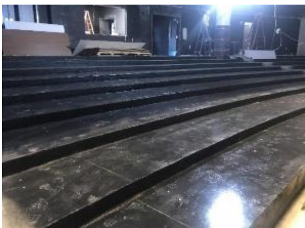
Upper seating concrete area has been stained. Seating layout work is in progress
