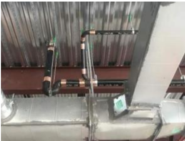
Cast iron drain lines are being installed below the mech. mezzanine deck. Mechanical duct joints are being sealed.
