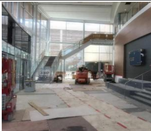
Nearing completion of painting and installation of railing glass panels.
