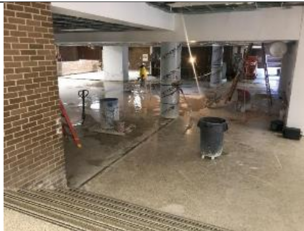
Terrazzo flooring is being polished in the lower Commons area.
