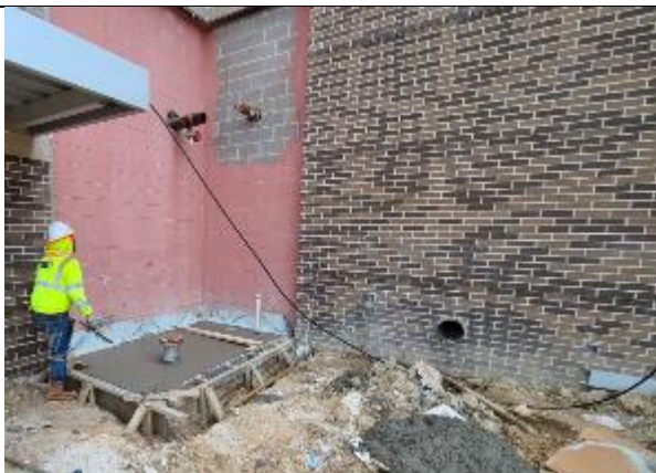
Fire Riser room pour back is complete.
