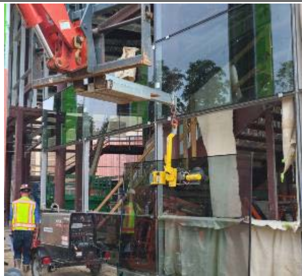
Curtain wall receiving glazing.
