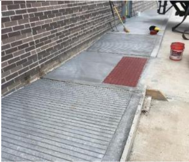
Accessible ramp and sidewalk have been poured along the Fire Lane.
