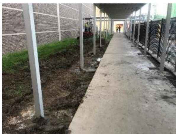
Prepping grading for the extension of the sidewalk work.
