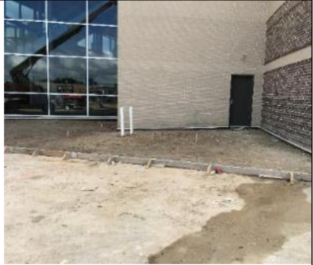
The sidewalk area is being prepped for concrete placement.
