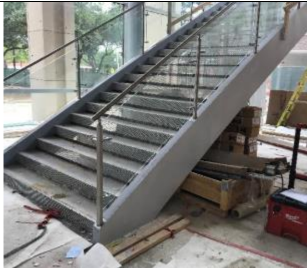
Monumental stair stringers are being filled and painted.
