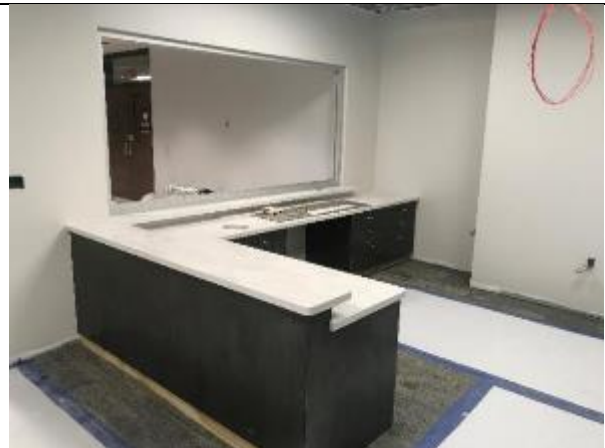
Casework has been installed. Carpet work has been completed and is awaiting base. Fire alarm wiring and installation is in progress.
