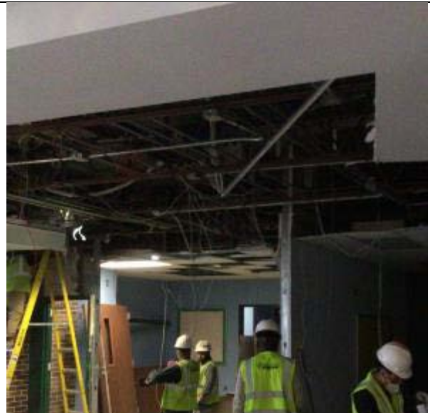
Plaster ceiling demo progress in corridors in existing campus.
