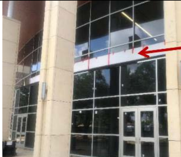
Low roof above entry aluminum panel work is being completed.
