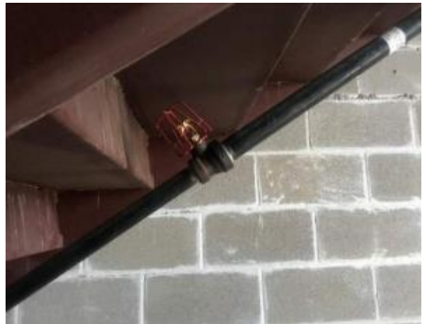
Fire sprinkler lines have been installed under the stair to the mezzanine
