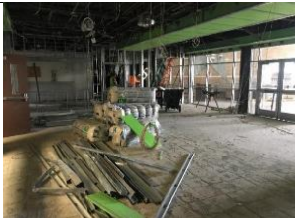
Demolition work has been completed and interior stud partitions in Area A are on-going.
