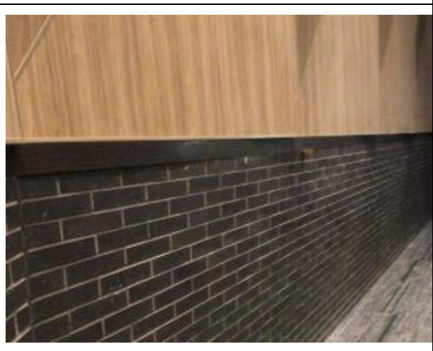
PLam sill under PSI panels inside Auditorium.
