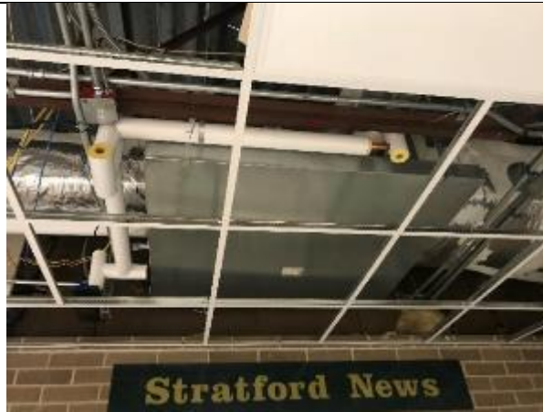
Condensate lines are being insulated for the new plenum mounted HVAC units.
