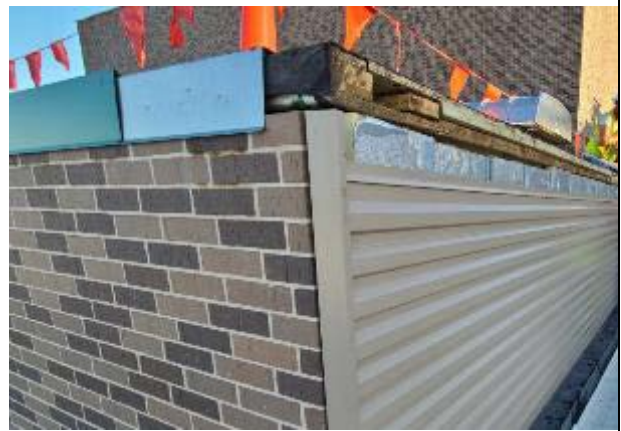
Metal panels installed at addition and existing intersection.
