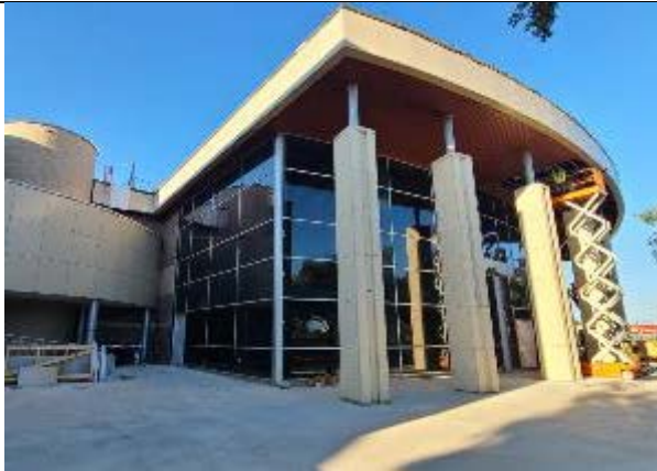
Exterior wood-look ceiling panels being installed at the canopy.
