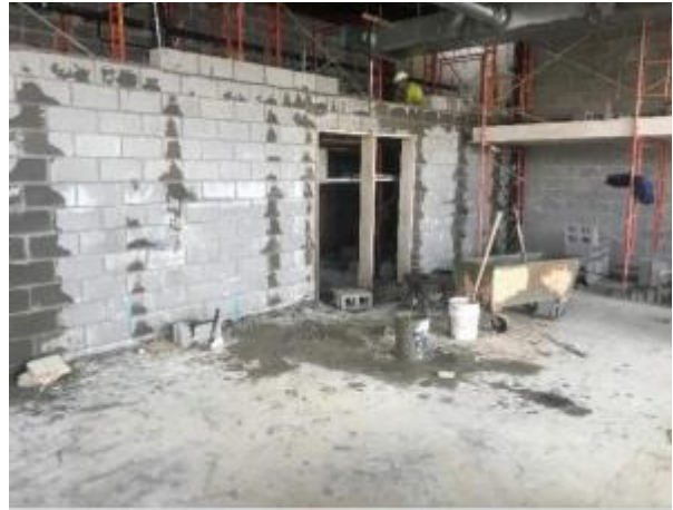
CMU block is being placed along corridor B126.
