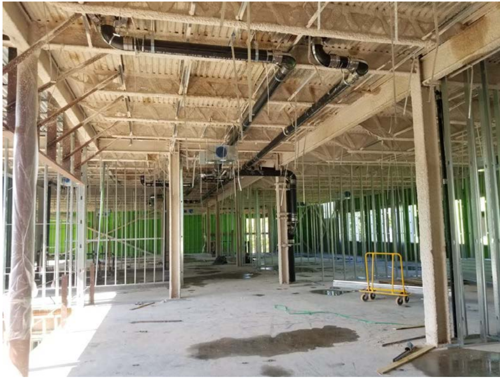
Second Floor interior framing and fireproofing
