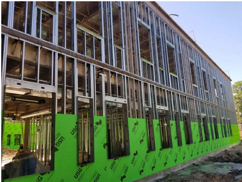
Exterior Framing and Sheathing
