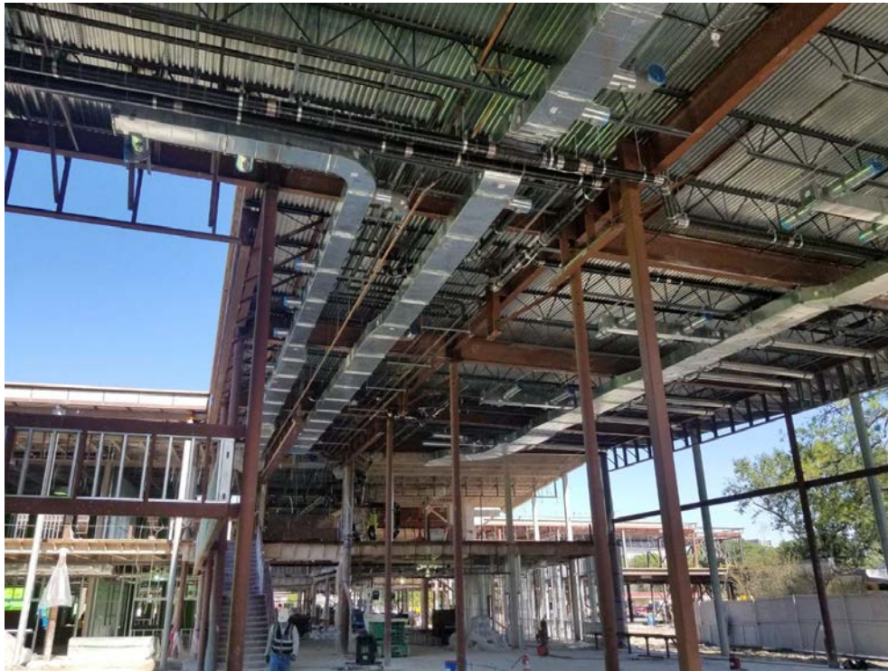
Ductwork and Piping in Main Corridor
