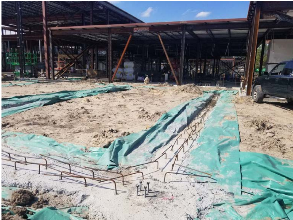
Grade Beams at Covered Play Slab
