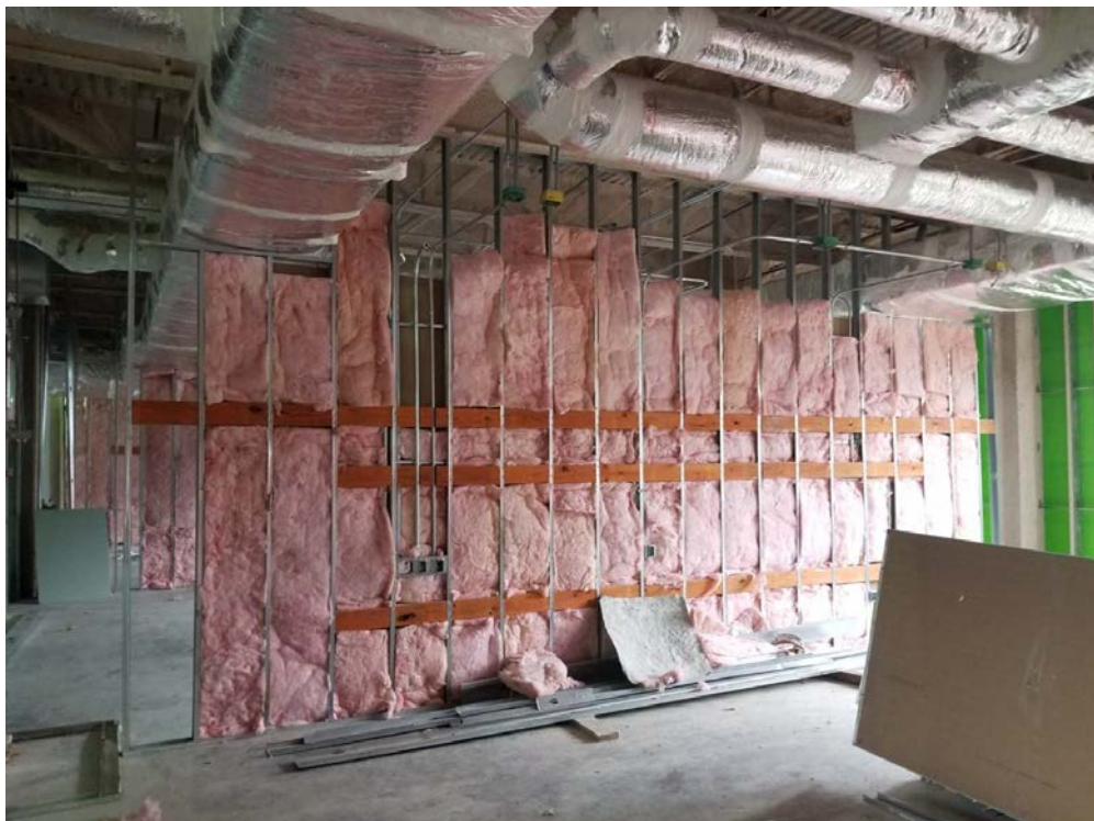
Classroom Wall Framing with Insulation
