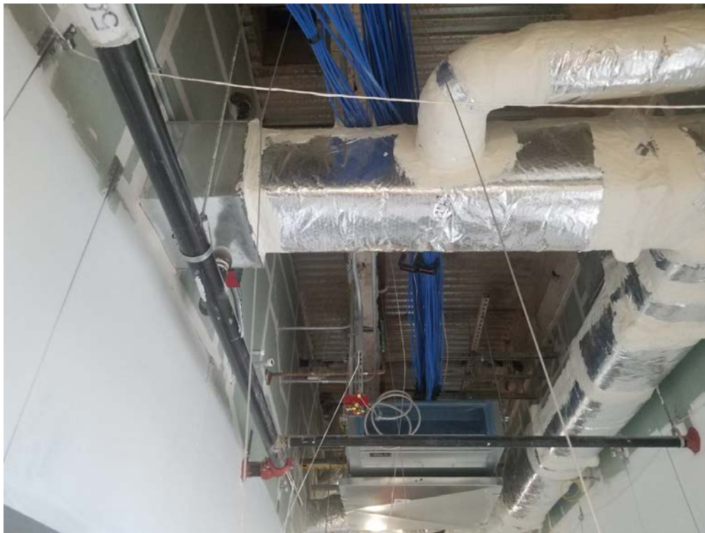
Ductwork and Data Cabling at Admin Corridor
