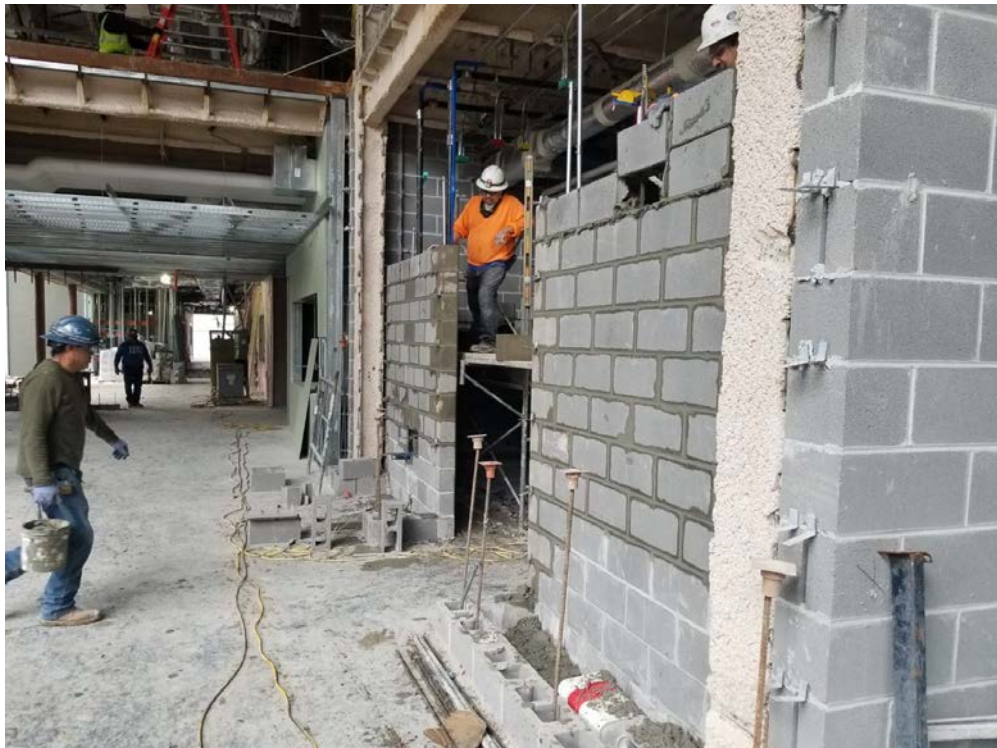
CMU Wall Install at Restroom near Dining
