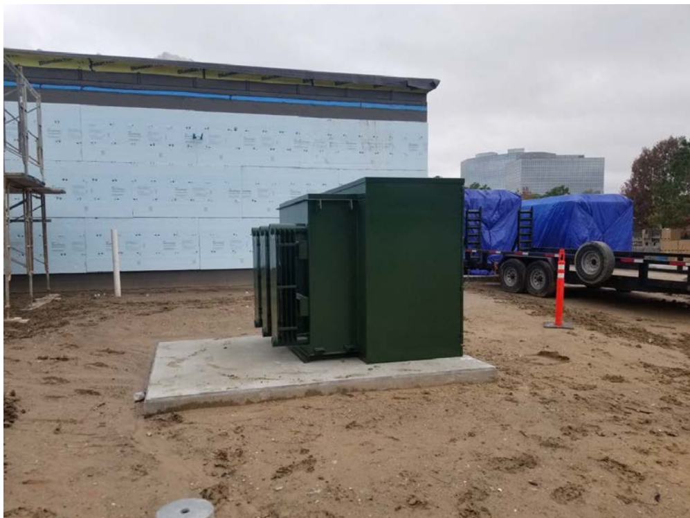
Center Point Transformer Set on Pad
