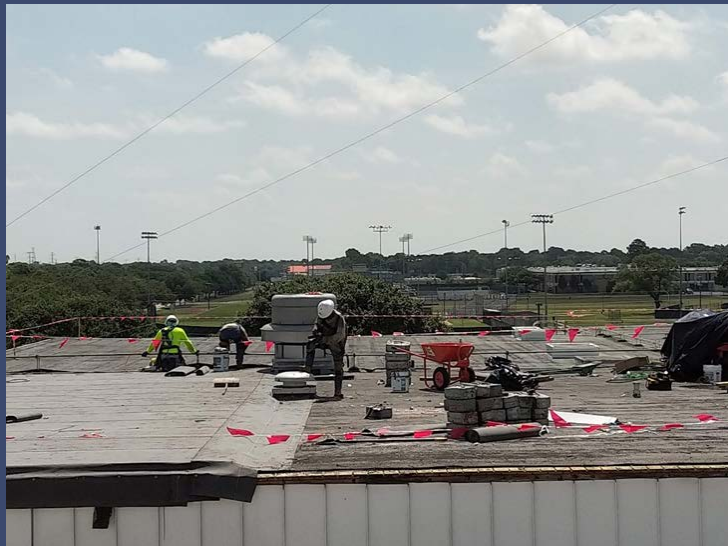
Installation of new roofing overlay
