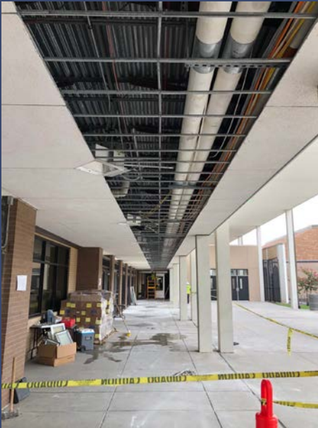
Section of Mechanical Pipe Replacement at Front of the Campus
